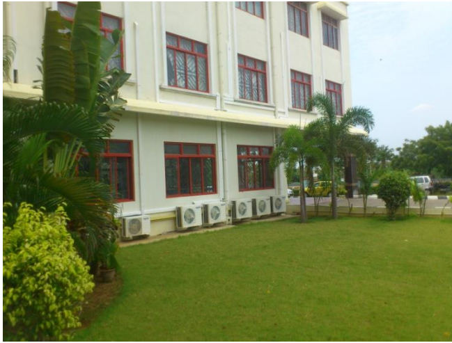
North Western side
